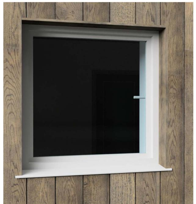
Use silicone behind the fascia boards where they meet the window to prevent the passage of any water getting through.
